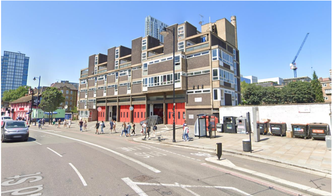
Figure 49: Shoreditch Training Centre
